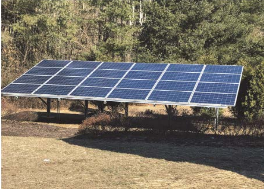
Figure 5-66 (RE5) Ground-Mounted PV Installation Photograph by Paul Torcellini, NREL 55603
