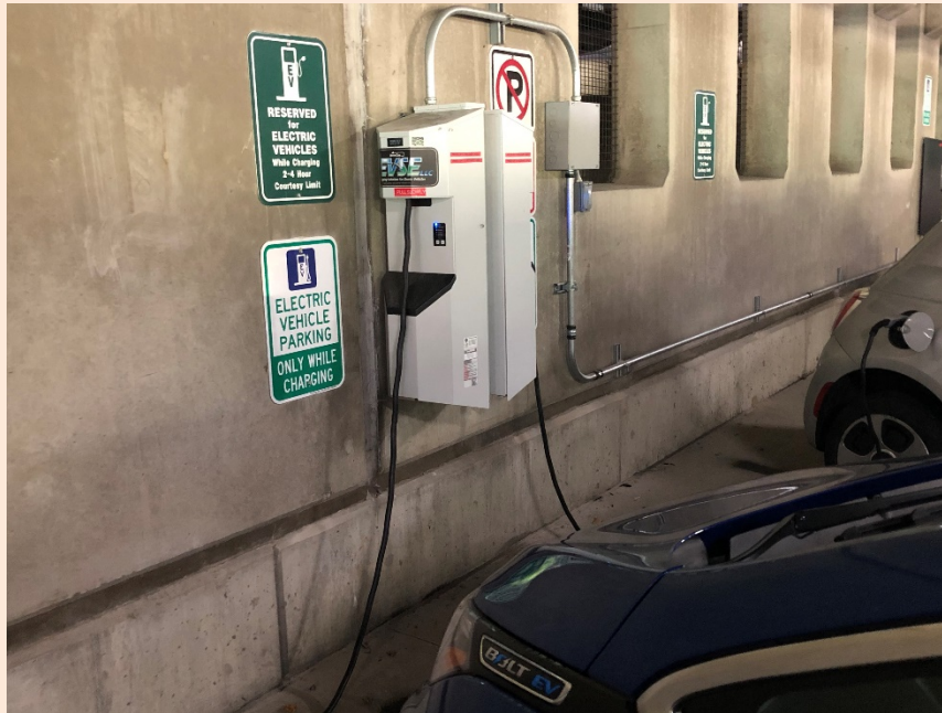
EV Charging Station
